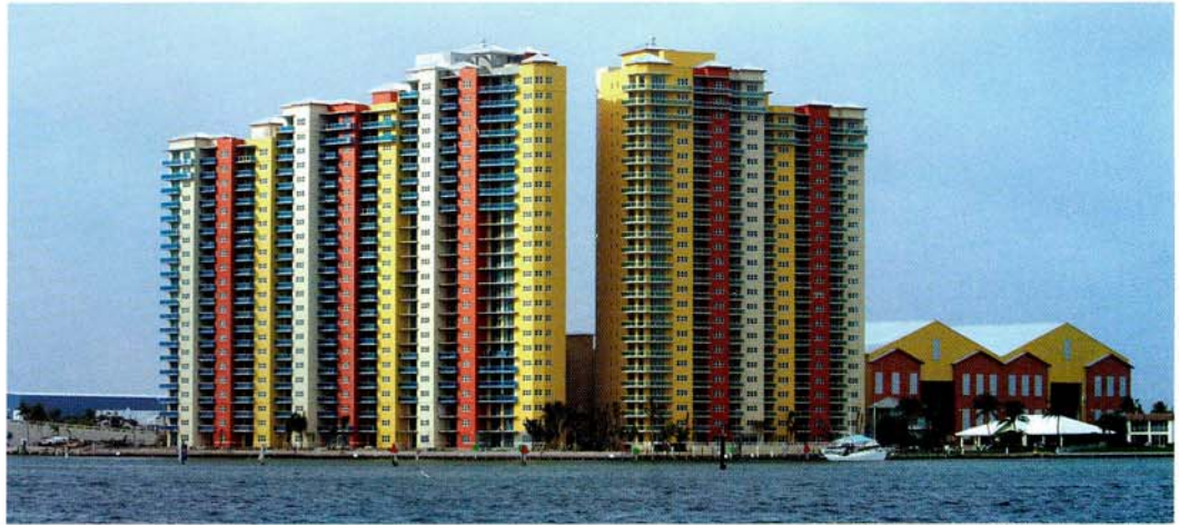
Photo courtesy of BCArchitects AIA, Inc.
